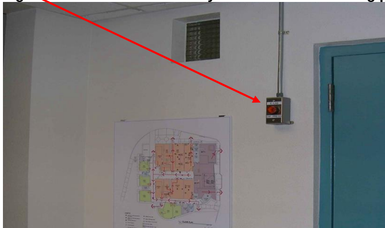
Example of amber light located in central hallway for differential building pressure issues
