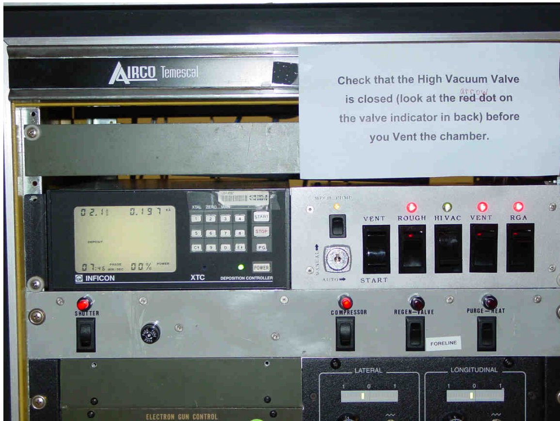
Figure 2 Inficon Thickness Monitor, Valve Control Panel and Shutter Switch
